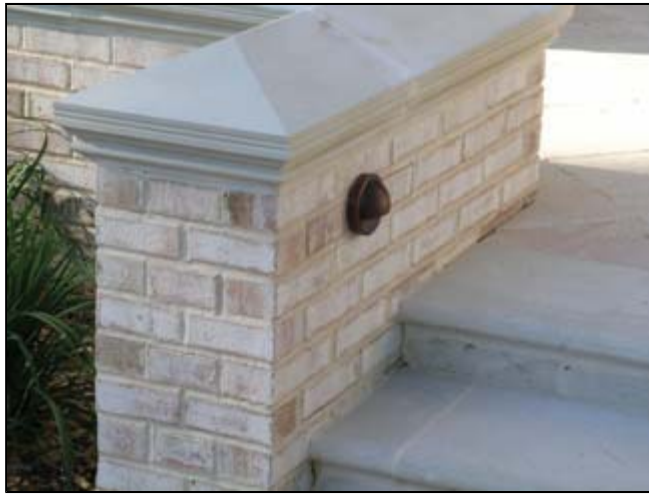
This surface-mounted puck light guides visitors up the steps leading to the home's front door. The trade name for this fixture is Gemini.
