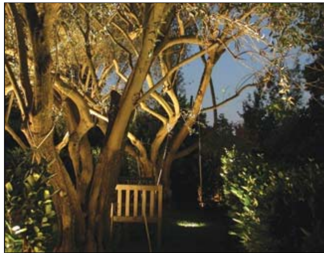
A close up of an olive tree uplift by well lights. The Apollo fixtures are flush with the grass and can be mowed over without any damage to the stainless steel socket and solar lenses. A cover is always used when the fixture is used in a planting bed to prevent debris from falling inside the fixture and touching the lamp, which could possibly cause a fire.
